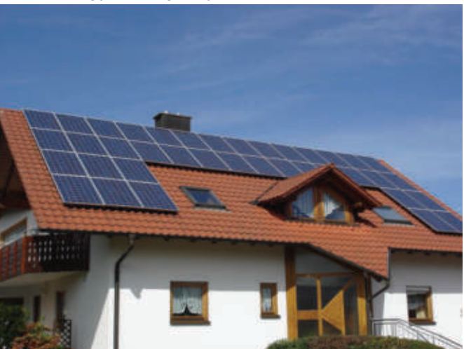
▼ Germany Integrated Photovoltaic Energy Storage System
